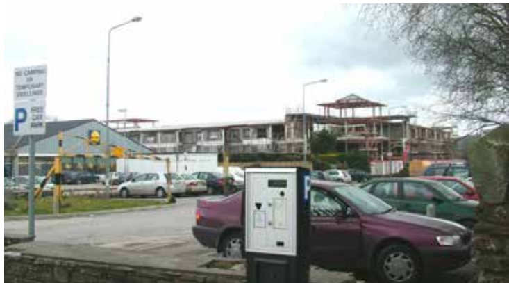
Dunn's Stores Macroom under construction in 2007.
