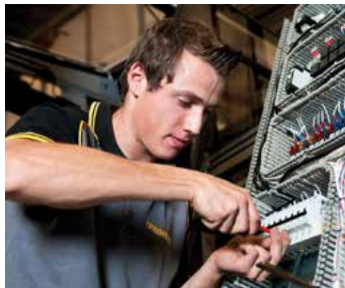
An electrical apprentice wires a crane's switchgear
