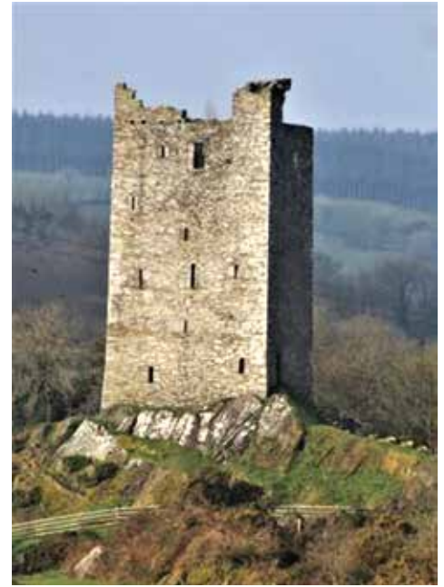
Carrigaphoooca tower house
