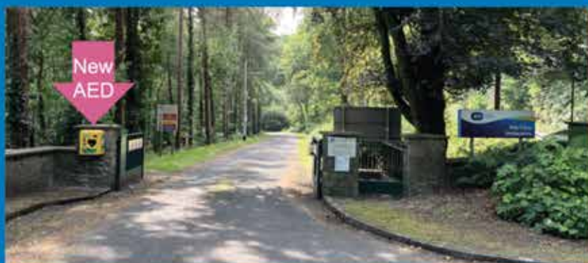
Overview of New AED at Entrance to Inniscarra Generating Station (P31 RC93)
