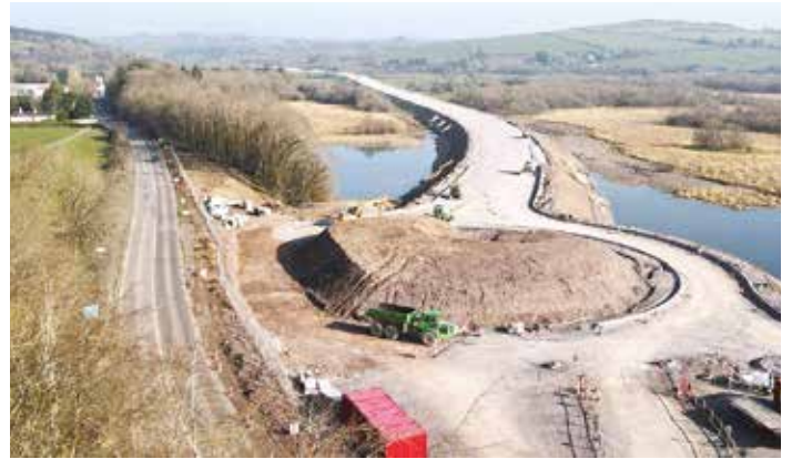
The new roundabout at Coolcower on the 27-3-22. Pic Peter Scanlan
