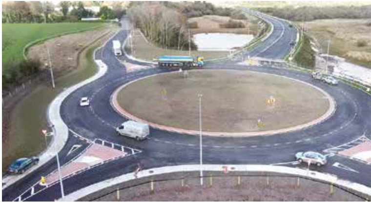
The new roundabout at Coolcower. Pic Peter Scanlan
