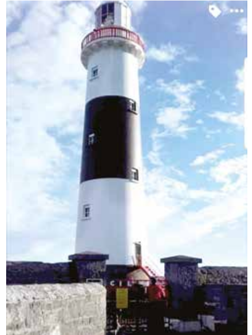
The Lighthouse at Fordurris Point on Inisheer.
