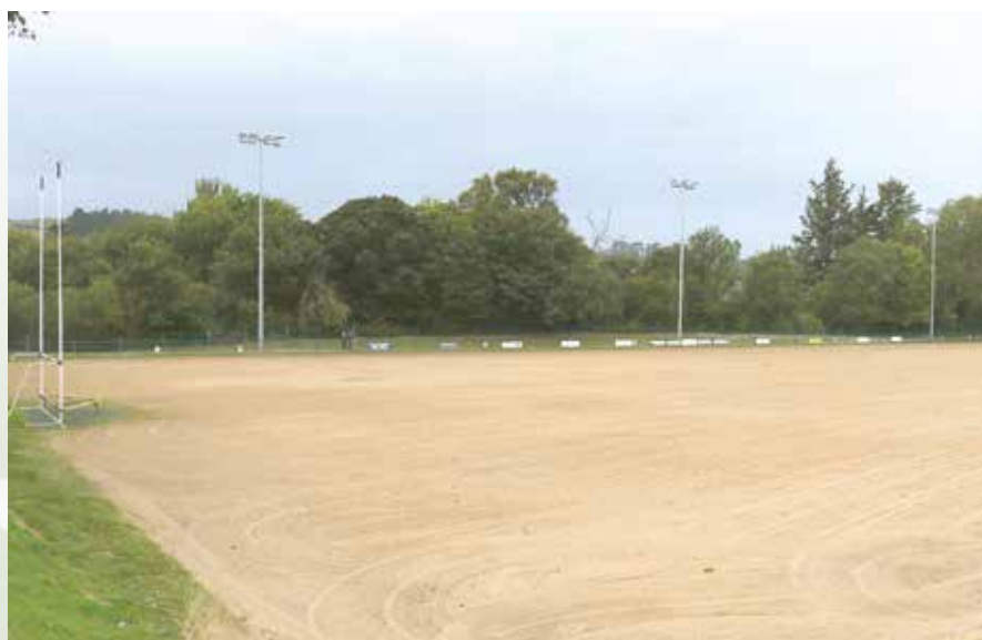
(Im)perfect pitch; Bishop McGegan Park, Castle Grounds, Macroom is being improved with extra drains, sanding and re-seeding/re-sodding. (C. Kelleher.)
