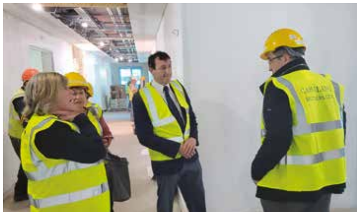
New building under construction at Macroom Hospital. Mary Butler, Aindrias Moynihan.
