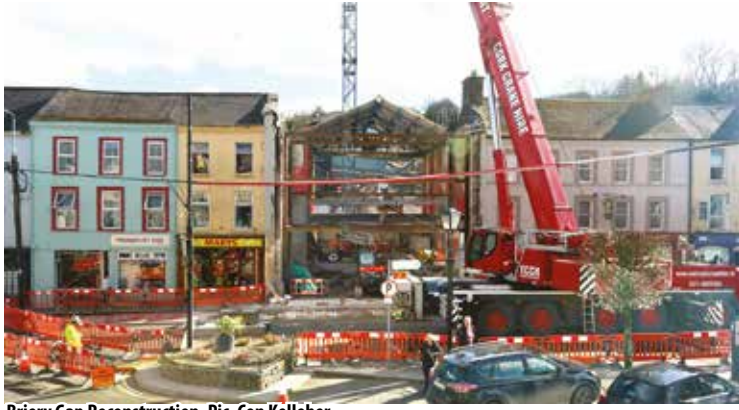
Briery Gap Reconstruction. Pic. Con Kelleher
