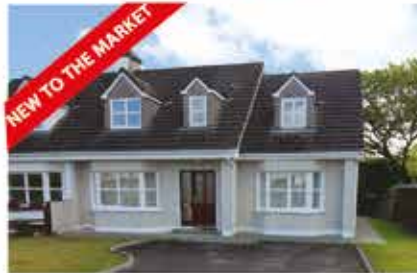
37 SULLANE WEIRS, MACROOM, CO. CORK, P12T627
