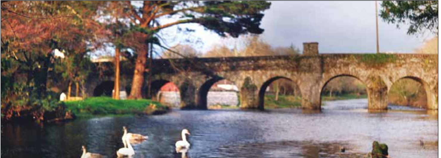
Castle Street Bridge Macroom, in the 1990's. © Peter Scanlan
