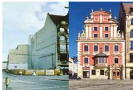
Before/After: Building restoration, Wroclaw, Poland
