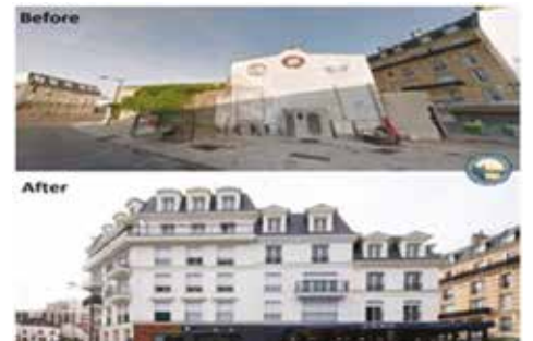
Before/After: Building restoration, Paris, France
