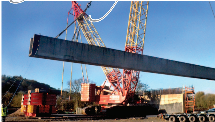
The Building of the Longest Bridge in Ireland. This 155 tonne, 49.9 metres, first concrete beam for the longest bridge in Ireland was moved into position, to span the Launey River near Bealick Mill on the Macroom Bypass © Peter Scanlan
